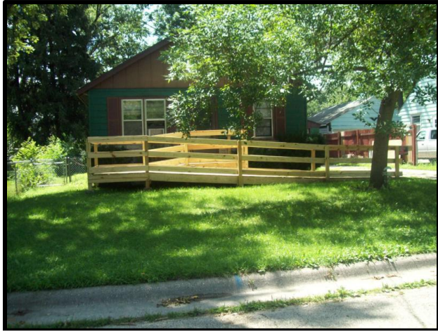
Pennsylvania Avenue Ramp
